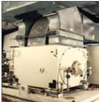
This 3500HP, 3/60/4000 Volt, 3600 RPM, TEFV horizontal motor is powering a pump on an oil pipeline.
